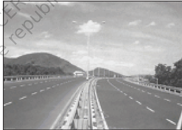
Fig. 8.3 : Dharmavaram Tuni National Highway, India
